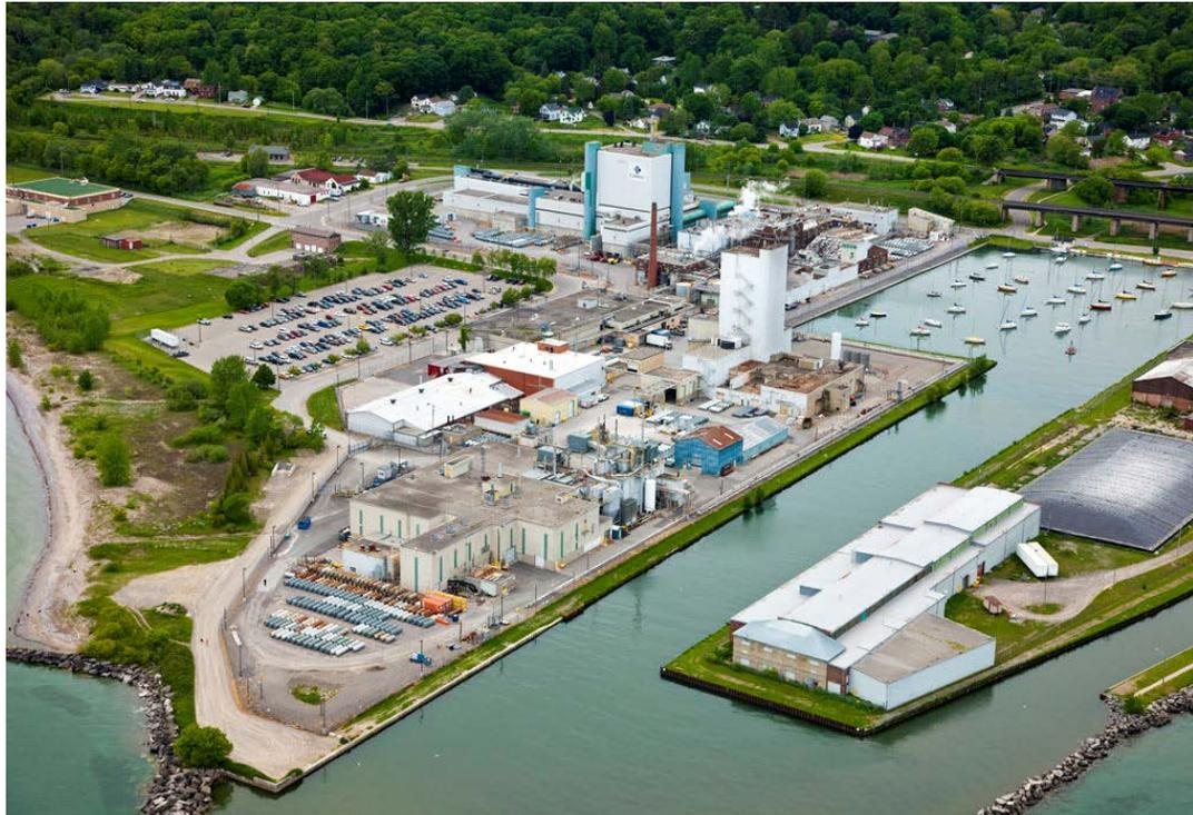
PHCF primarily converts uranium trioxide ( $\text{UO}_3$ ) powder produced by Cameco's Blind River facility into uranium dioxide ( $\text{UO}_2$ ) and uranium hexafluoride ( $\text{UF}_6$ ).  $\text{UO}_2$  is used in the manufacture of CANDU reactor fuel (natural uranium), while  $\text{UF}_6$  is exported for further processing before being converted into fuel for light-water reactors.
